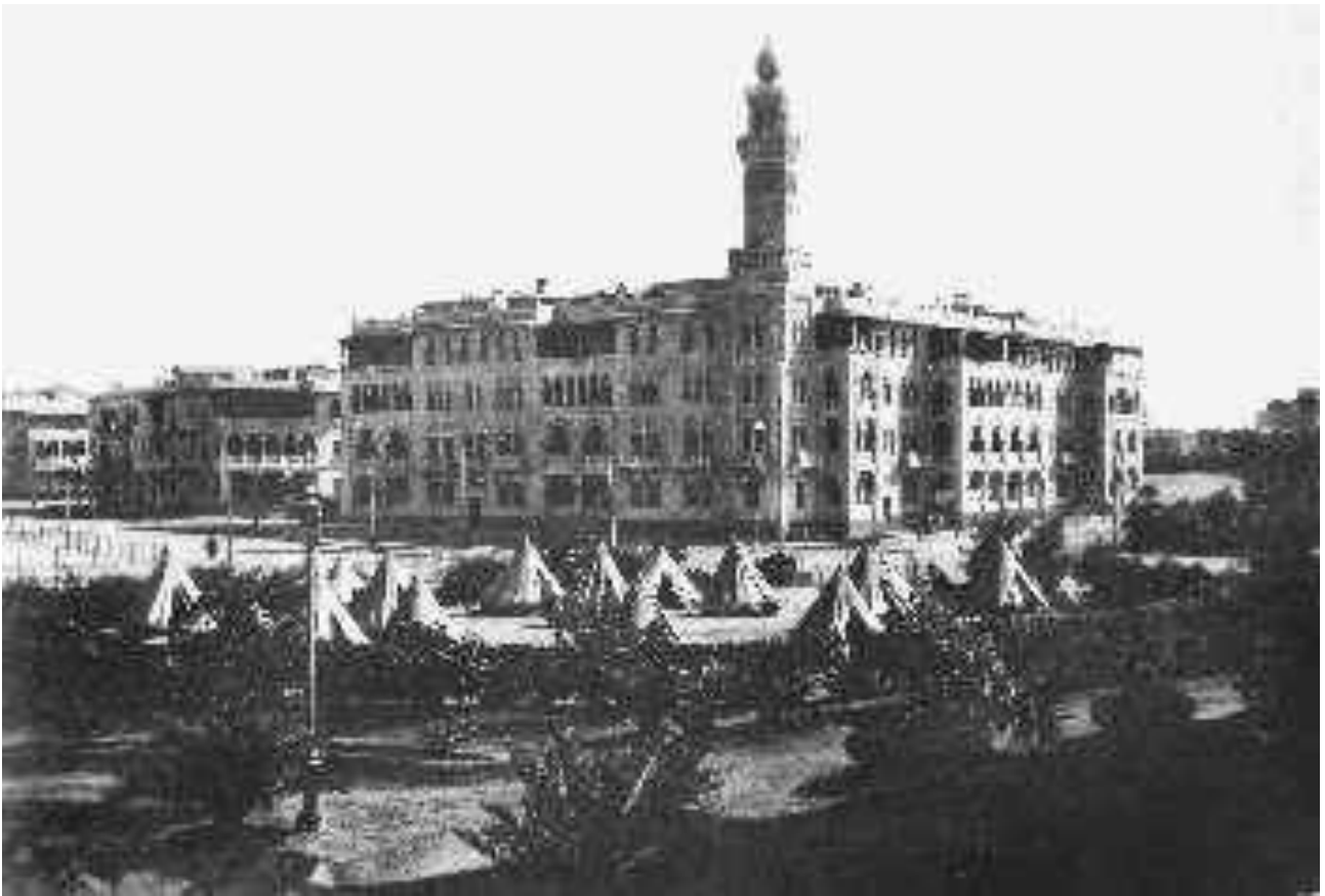
The Palace Hotel in Heliopolis, about 4½ miles west of Cairo, which had been re-purposed as the 1st Australian General Hospital.
